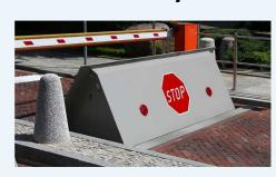
Integrate vehicle anti-ramming elements into the roads leading into your premises. Ensure these do not obstruct pedestrian movement/access.
